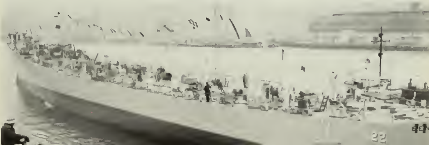
(11) Hull is floated out
